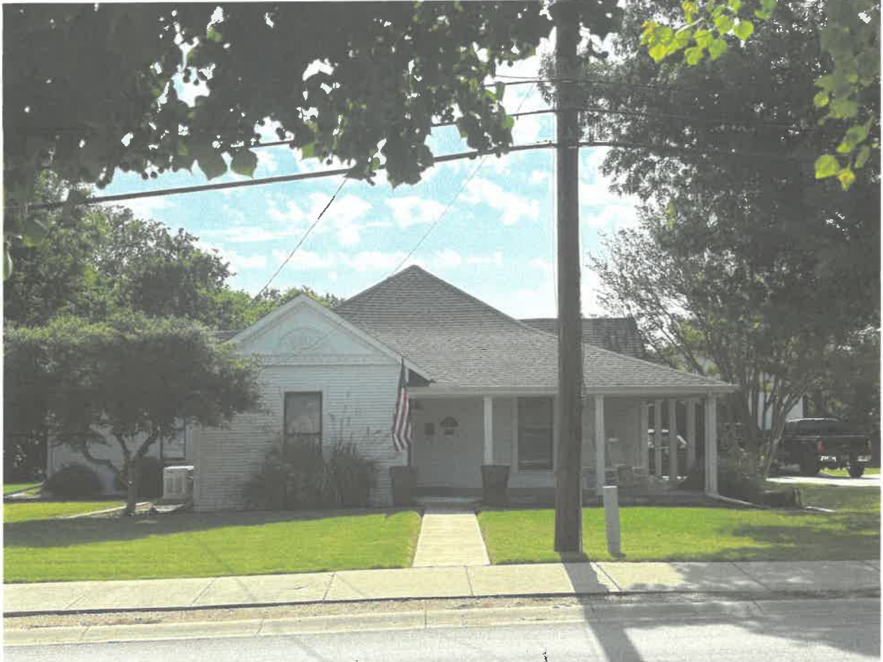
West (front) elevation from S Clark Street showing front porch, entry, and multiple double-hung windows. Front of house faces due west.
