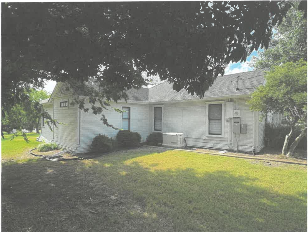
North side elevation showing additional double-hung windows and mechanical equipment.
