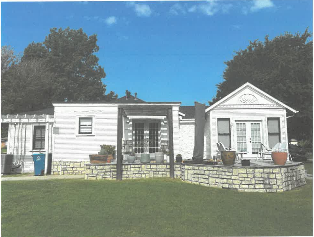
East (rear) elevation showing rear doors, windows, and stone patio area. Windows on this elevation are also proposed for replacement.
