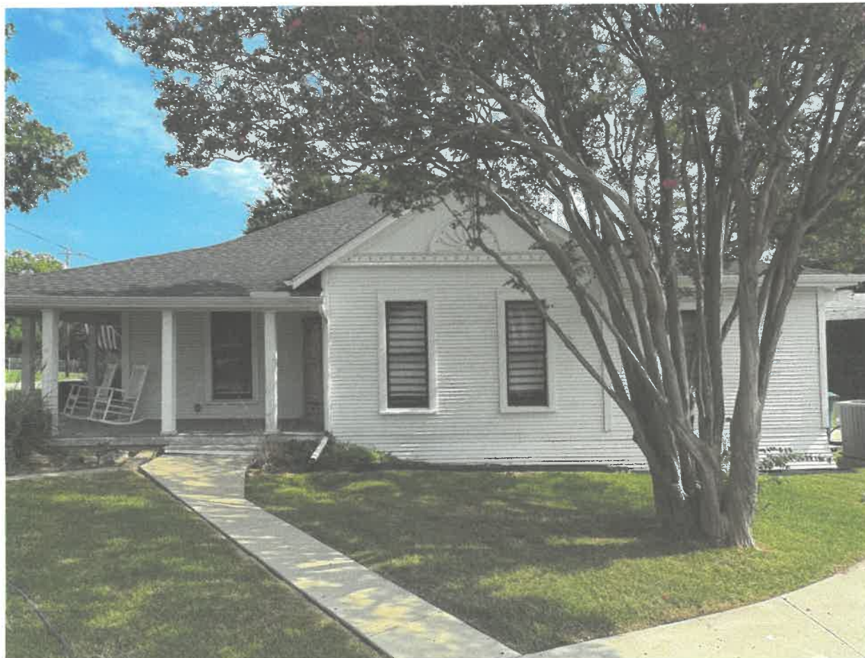
South elevation (front of house faces due west). Shows porch continuation and double-hung windows.
